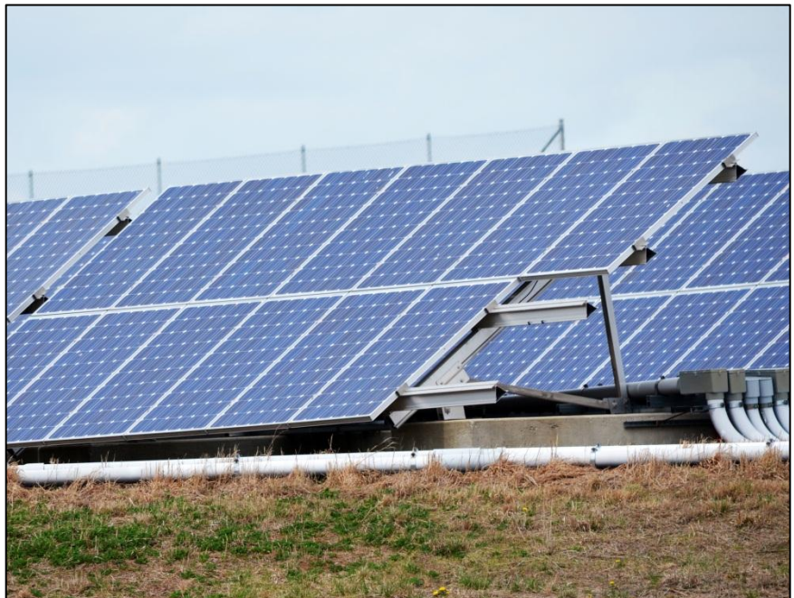
In 2010, the Commission approved an amended agreement that allowed solar panels to be built on the Stafford landfill.
